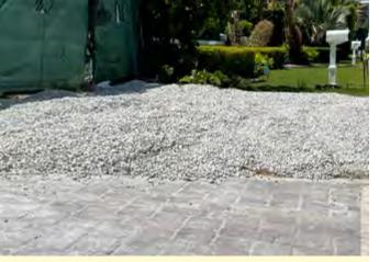
Allow for a gravel strip that is the lot width x minimum 15' from the valley gutter to accommodate construction parking.
